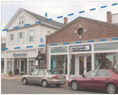
A: Similar Cornice Line and Roof Peak B: Similar Cornice Lines
