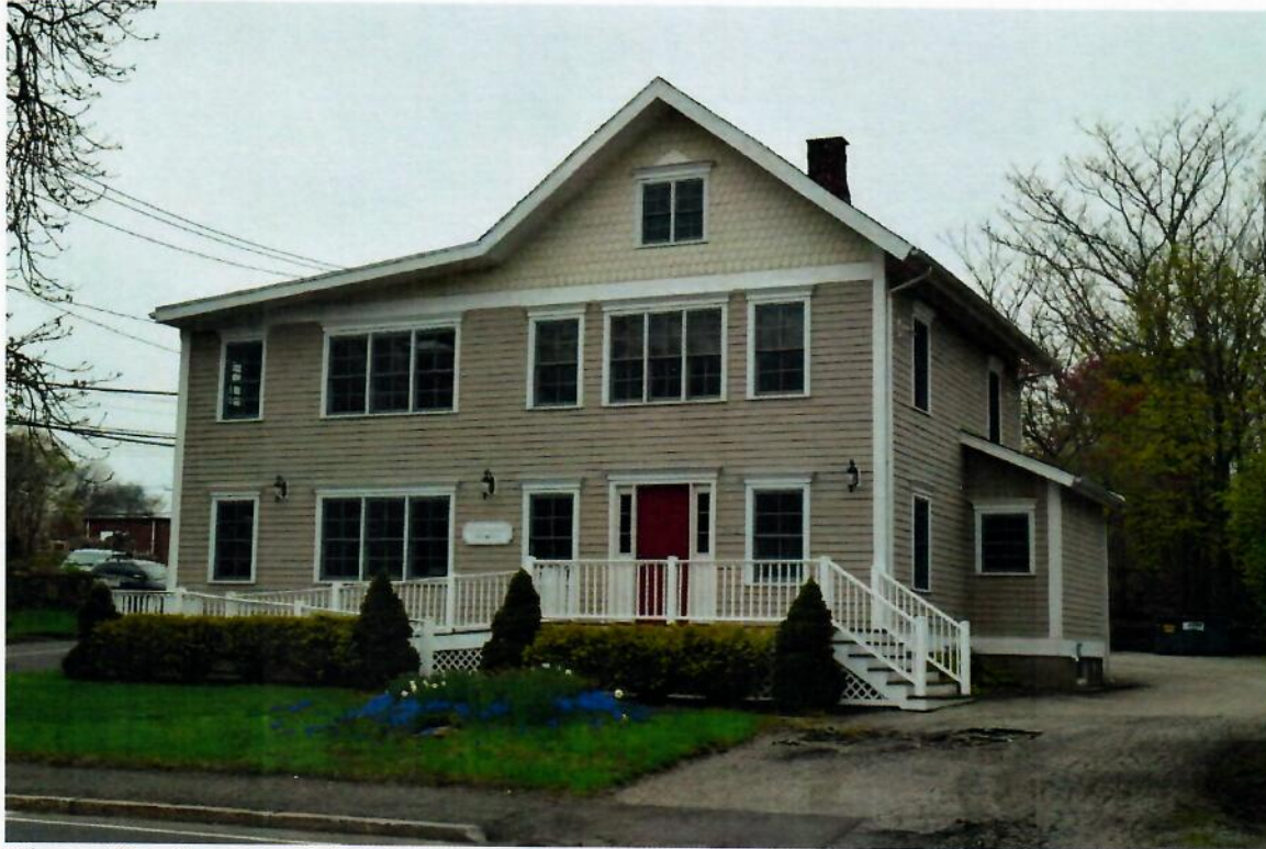
View of Southeast elevation.
