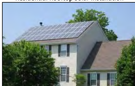
Residential Rooftop Solar Installation
