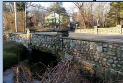
Greens Farm Road Bridge
